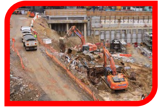
Additional construction disruption for basement dig
