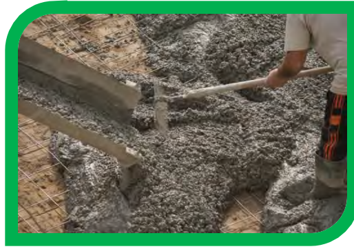
Reduced embodied carbon impact & construction programme
